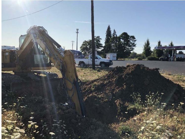
Test Pit Exploration Activity, TP-1
