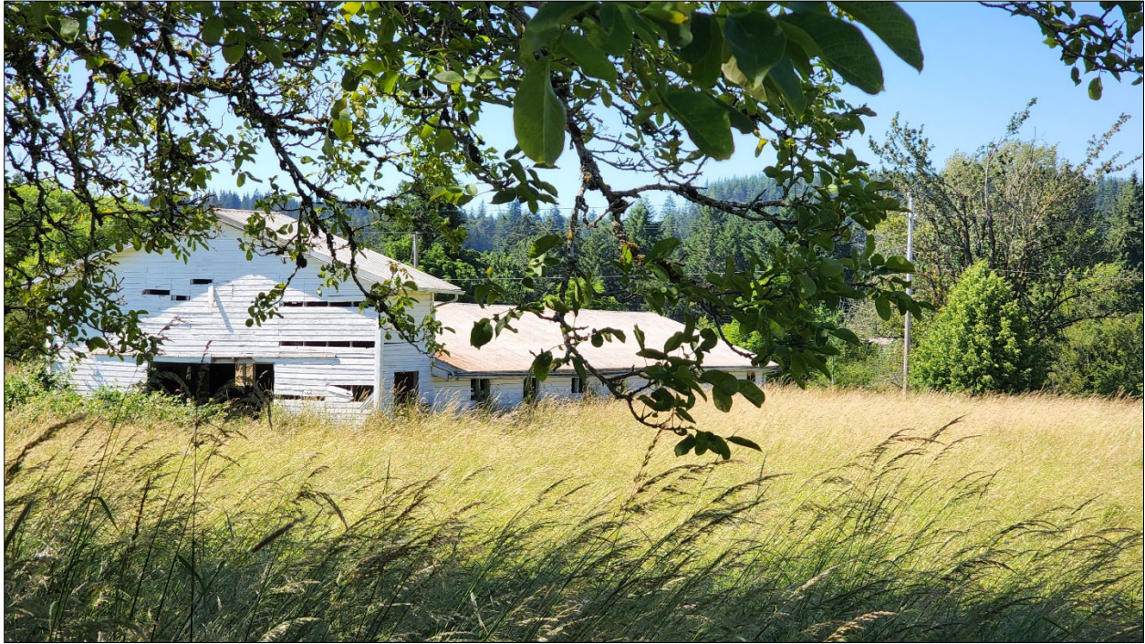
Photo 5. Barn in the central part of the site facing north.
