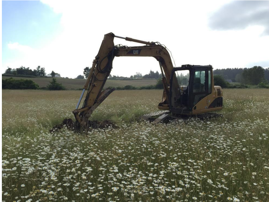
Conducting Test Pit Exploration in Southernmost Parcel
