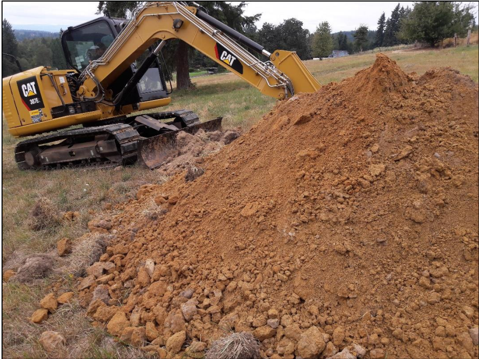
Conducting Test Pits, TP-10
