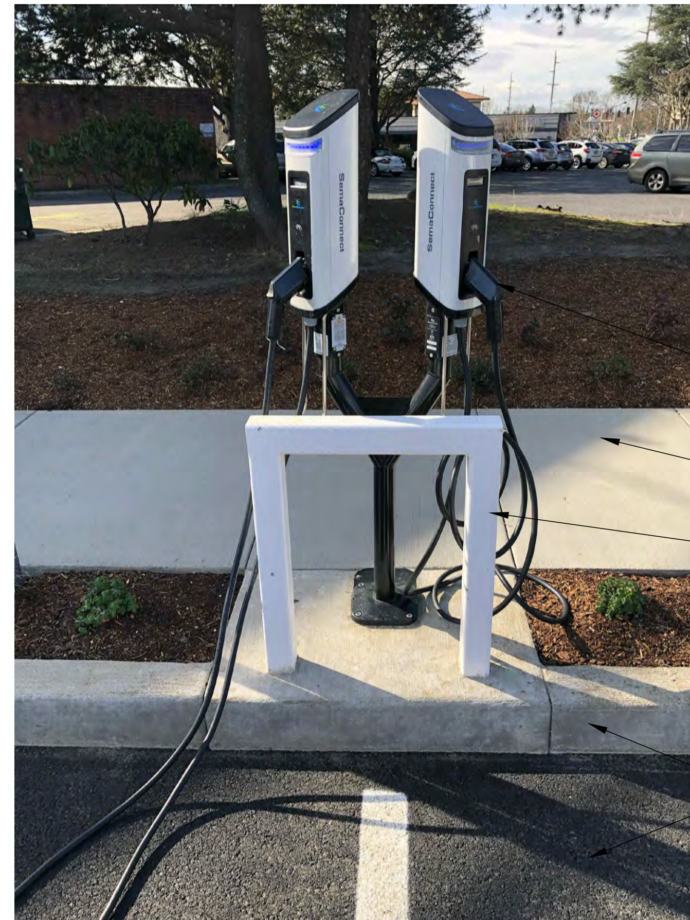
DUAL PARKING SPACE INSTALLATION
