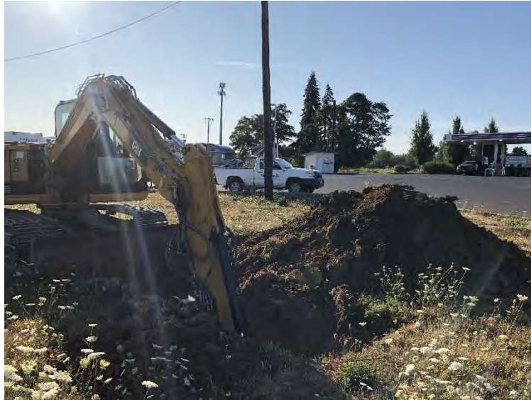
Test Pit Exploration Activity, TP-1
