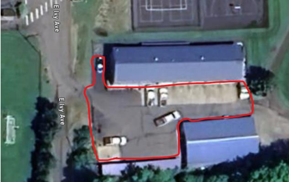
Lot 2. PW Shop: 291 Ivy Ave – approximately 12,000 square feet
