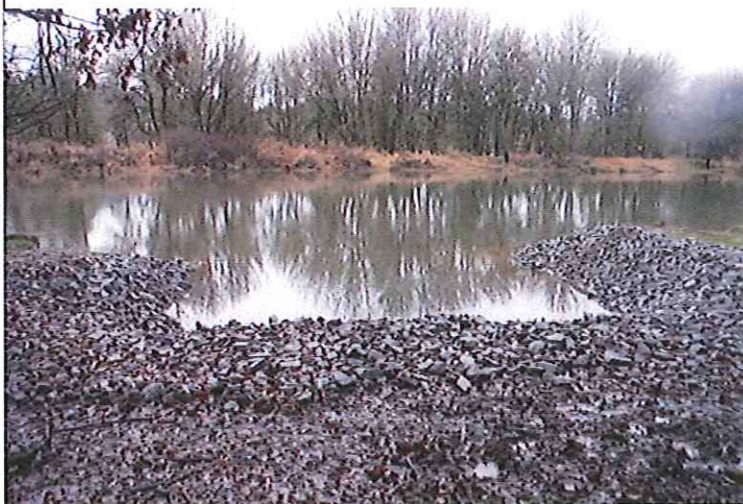
Storm Pipe Outfall Area
