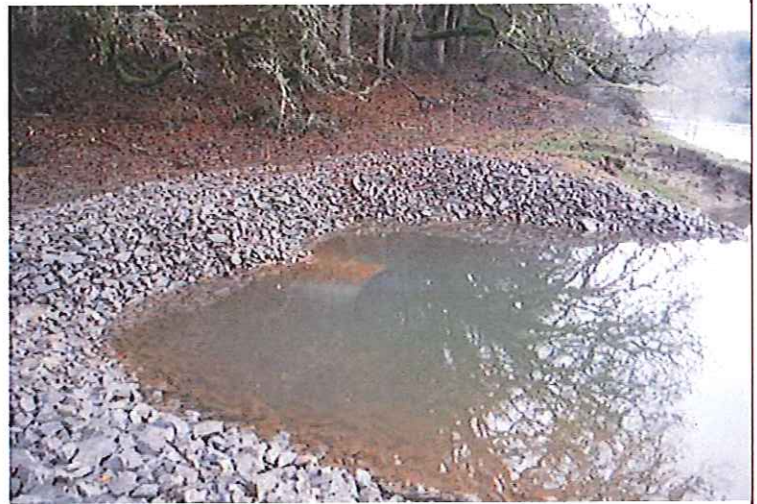
Submerged Outfall Pipe
