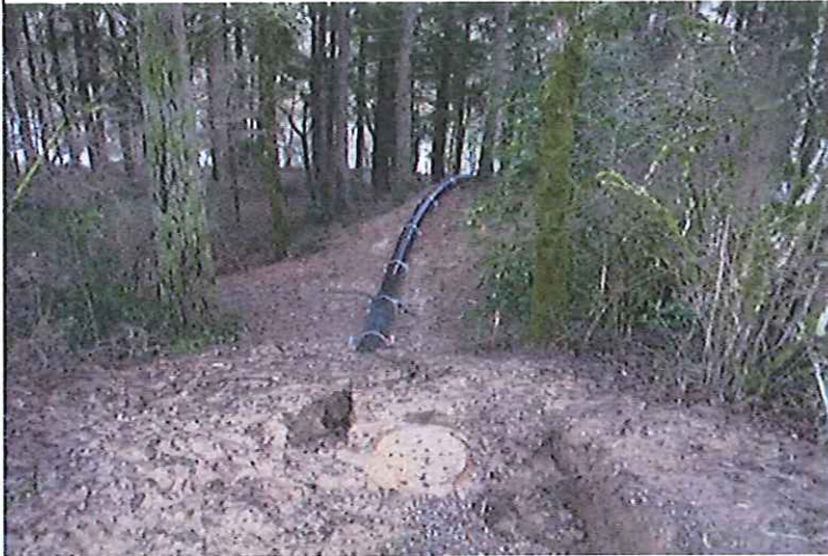
Upper Portion of Outfall Pipe
