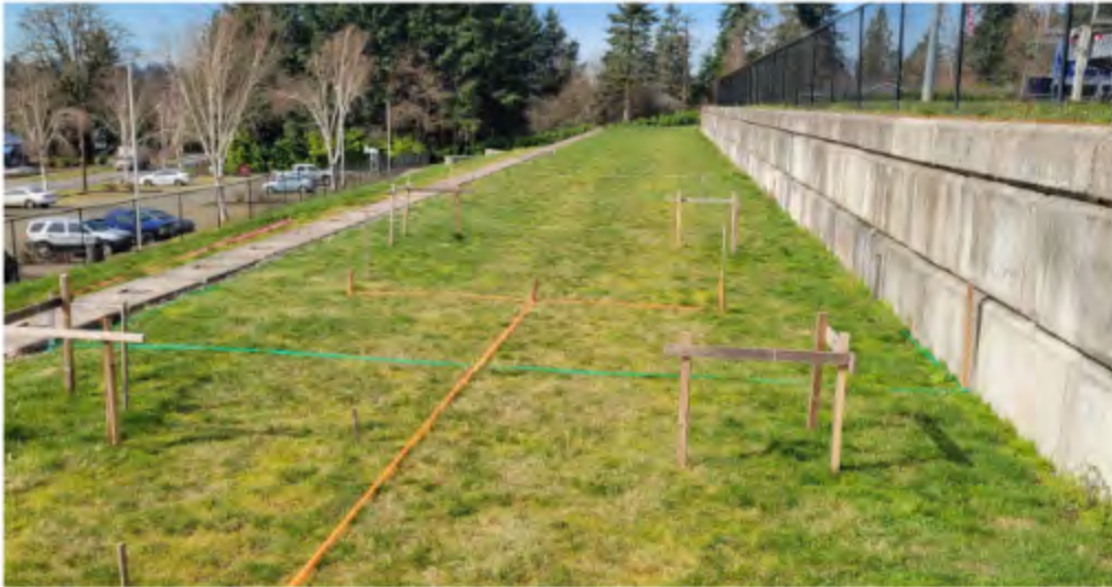
Photo 1. Project site – looking west across GreenShed site
