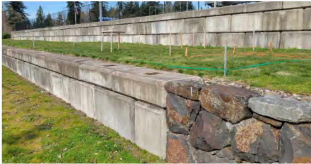
Photo 4. Project site – looking northwest at face of terraced Ultrablock Walls.
