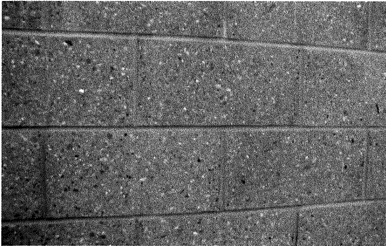
concrete polished CMU
