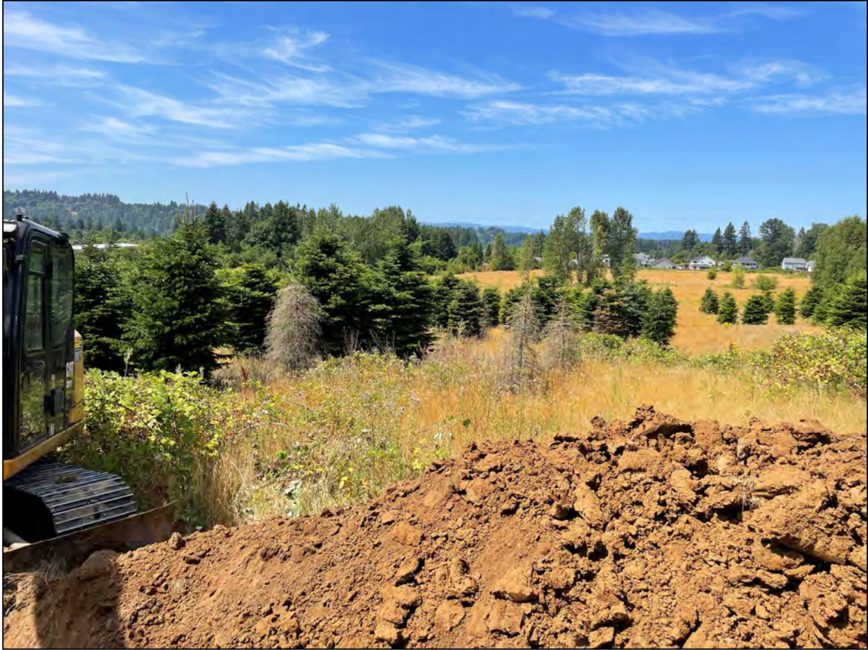
East Site View, Facing West
