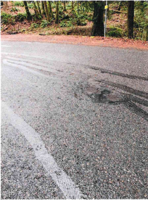
Crack Sealing of existing asphalt cracks
