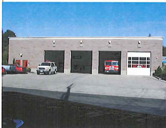
Equipment Bays at Fire Station
