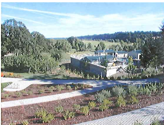
The Wastewater Treatment Plant South of Downtown
