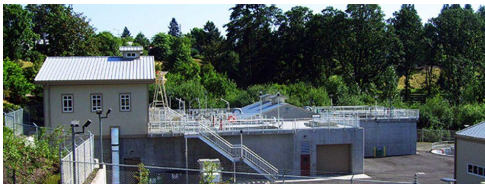
Figure 1: La Center Wastewater Treatment Facility
