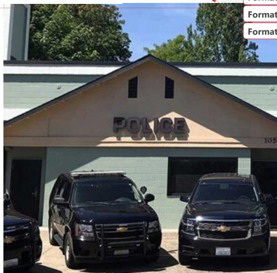
Figure 2: CCSO in La Center
