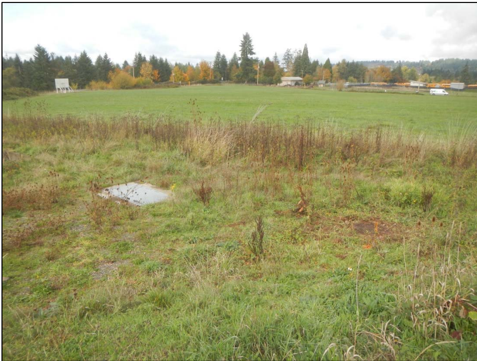
Photo 5. Manhole and steel vault. View is to the northwest.
