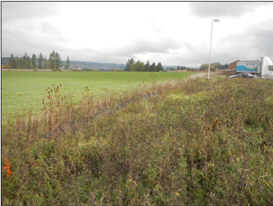
Photo 2. Eastern portion of study area showing silt fence at base of slope. View is to the east.
