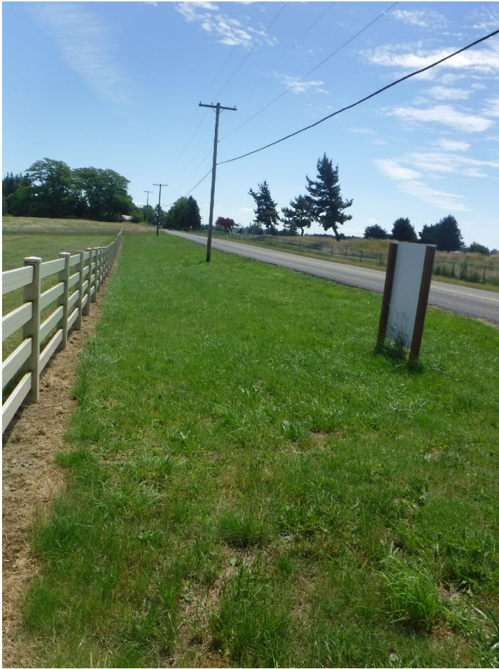
1. Maintained Right of Way - NW 11th Ave
