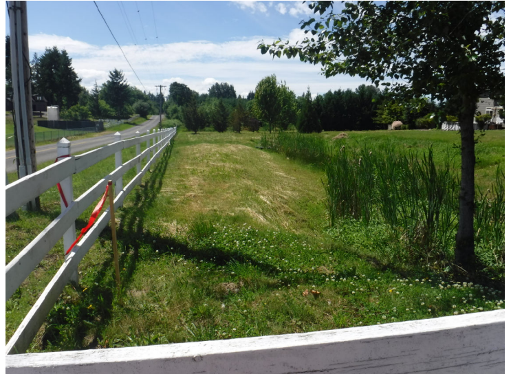
4. Proposed Utility Pole Location Near Stormwater Facility - NW 299th Street
