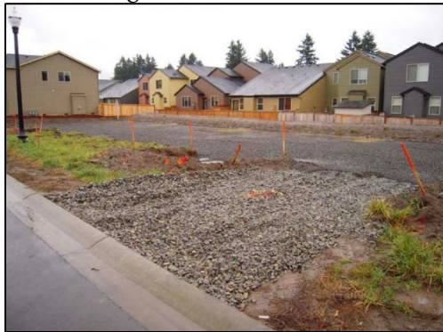
Figure 31: Small-scale Construction Entrance
