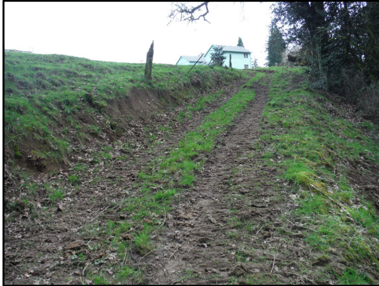
Figure 10. Photograph of the dirt roadway that has been cut into the hillside below the upper bench, looking south from middle bench.
