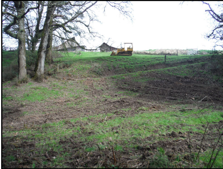
Figure 16. Photograph of upper and middle benches, looking east with roadway descending hillside from the right.
