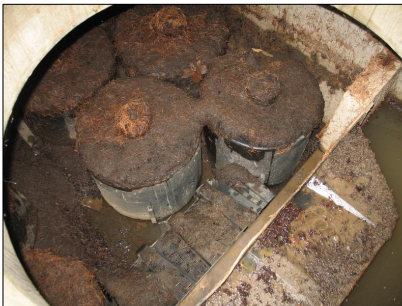
Media Cartridge Filter Vault with Accumulated Sediment
