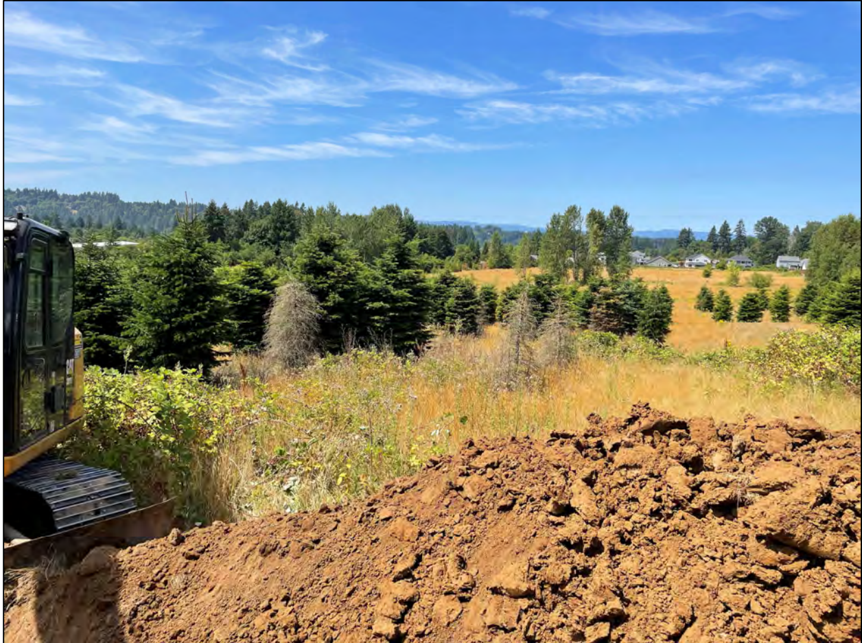
East Site View, Facing West
