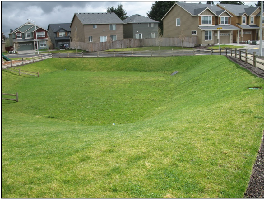
Example of a Manicured Detention Pond
