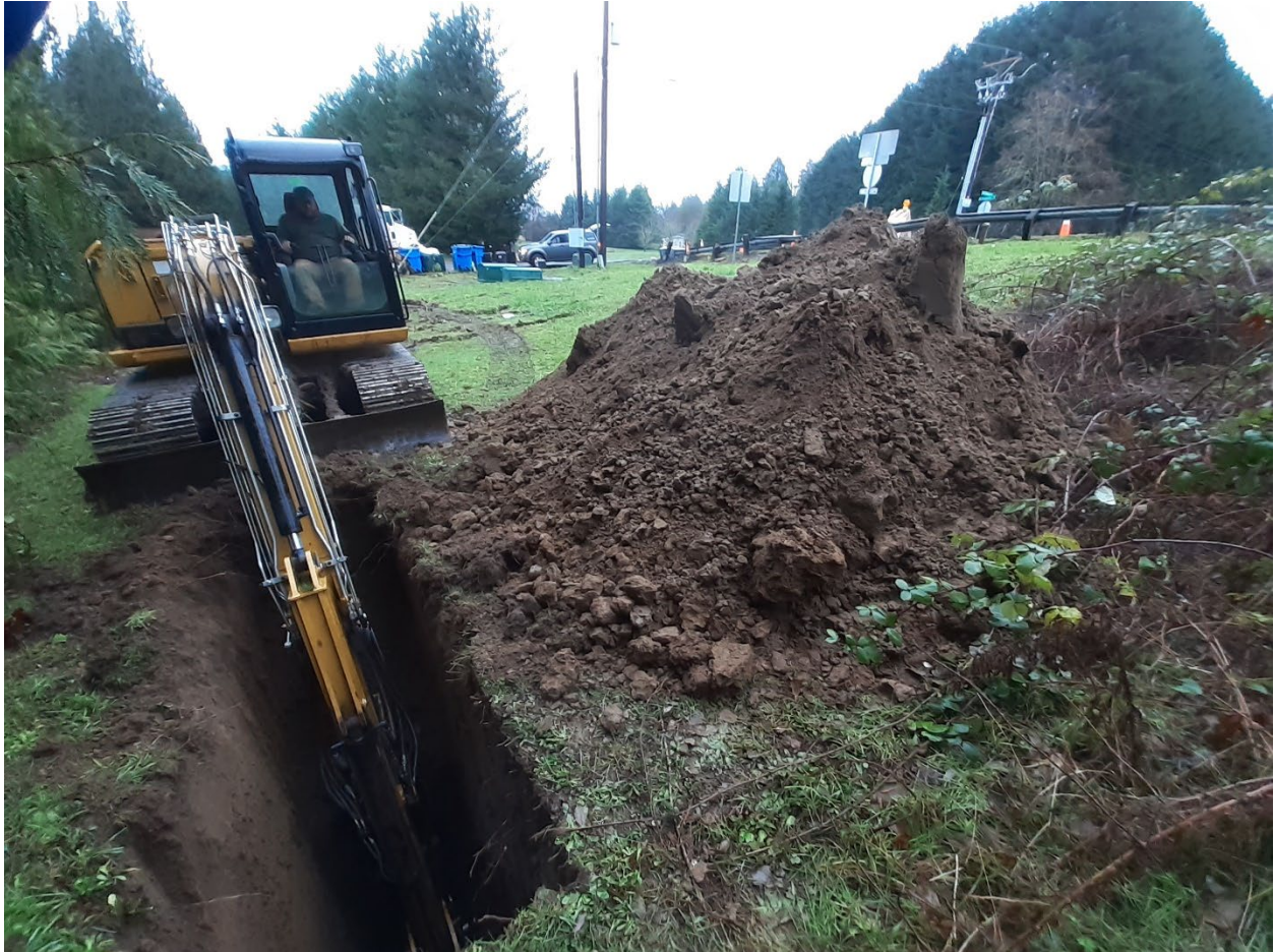
Western Site Area, Facing East
