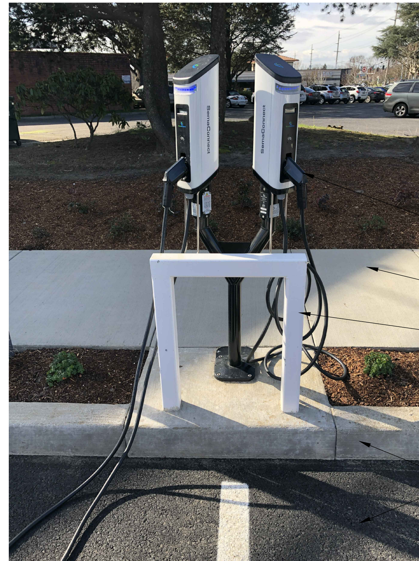
DUEL PARKING SPACE INSTALLATION
