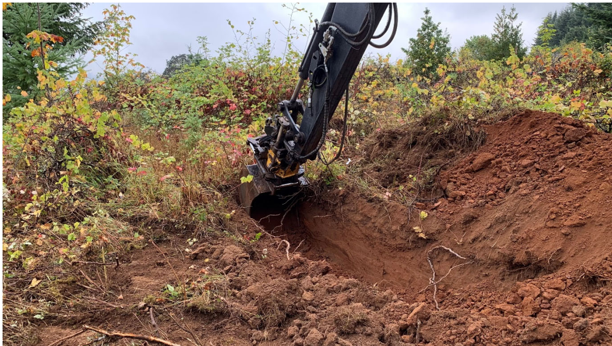
Photo 2. Excavating Test Pit 2.
