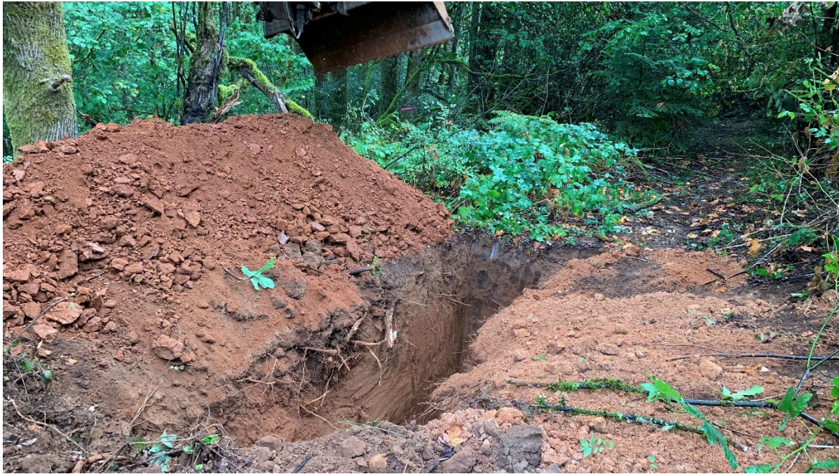
Photo 3. Excavation of Test Pit 3, just southwest of the gully.
