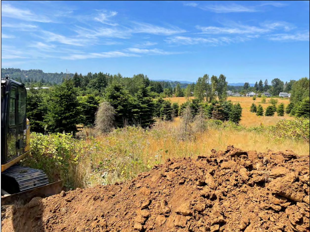
East Site View, Facing West
