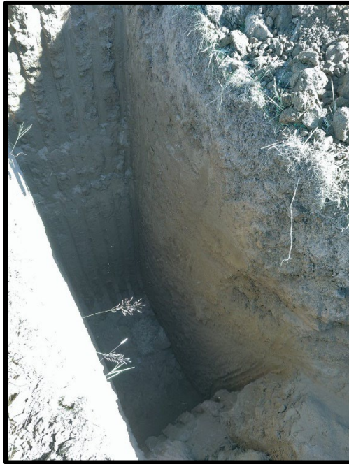
Test Pit, TP-8
