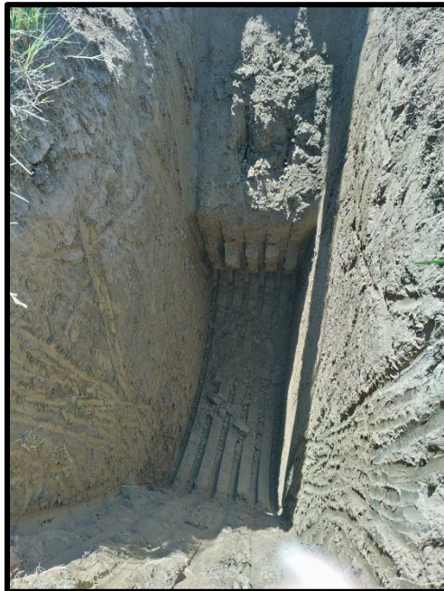
Test Pit, TP-7
