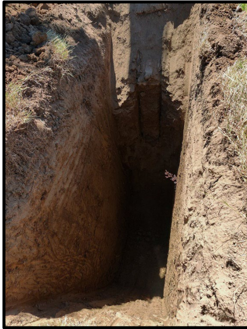
Test Pit, TP-1
