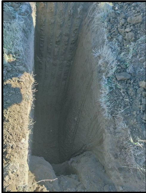
Test Pit, TP-2
