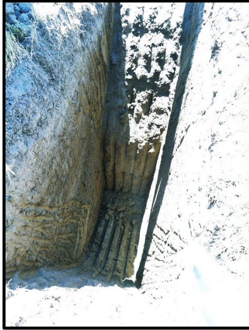
Test Pit, TP-4
