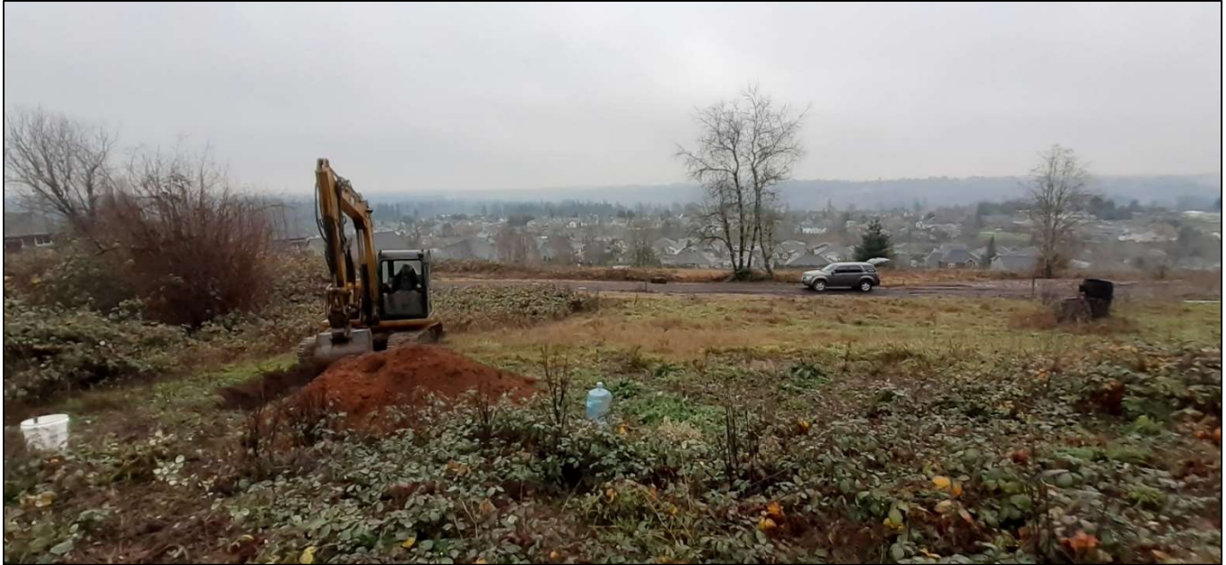
Conducting Test Pits, Looking South towards TP-1
