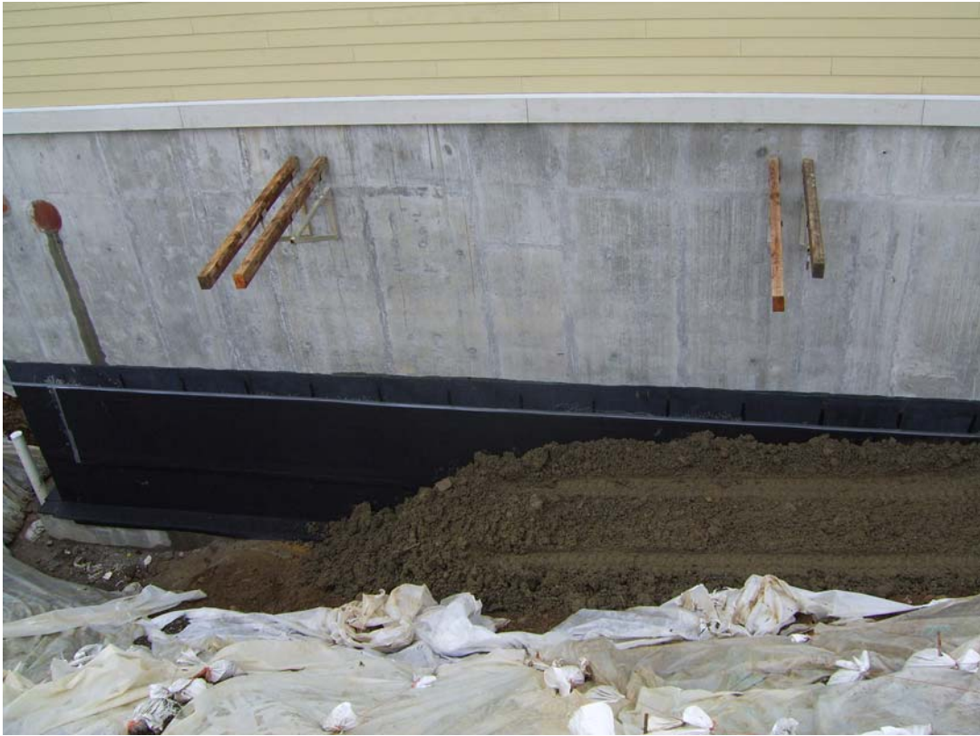
3/26/10 – Headworks exterior waterproof membrane and backfilling
