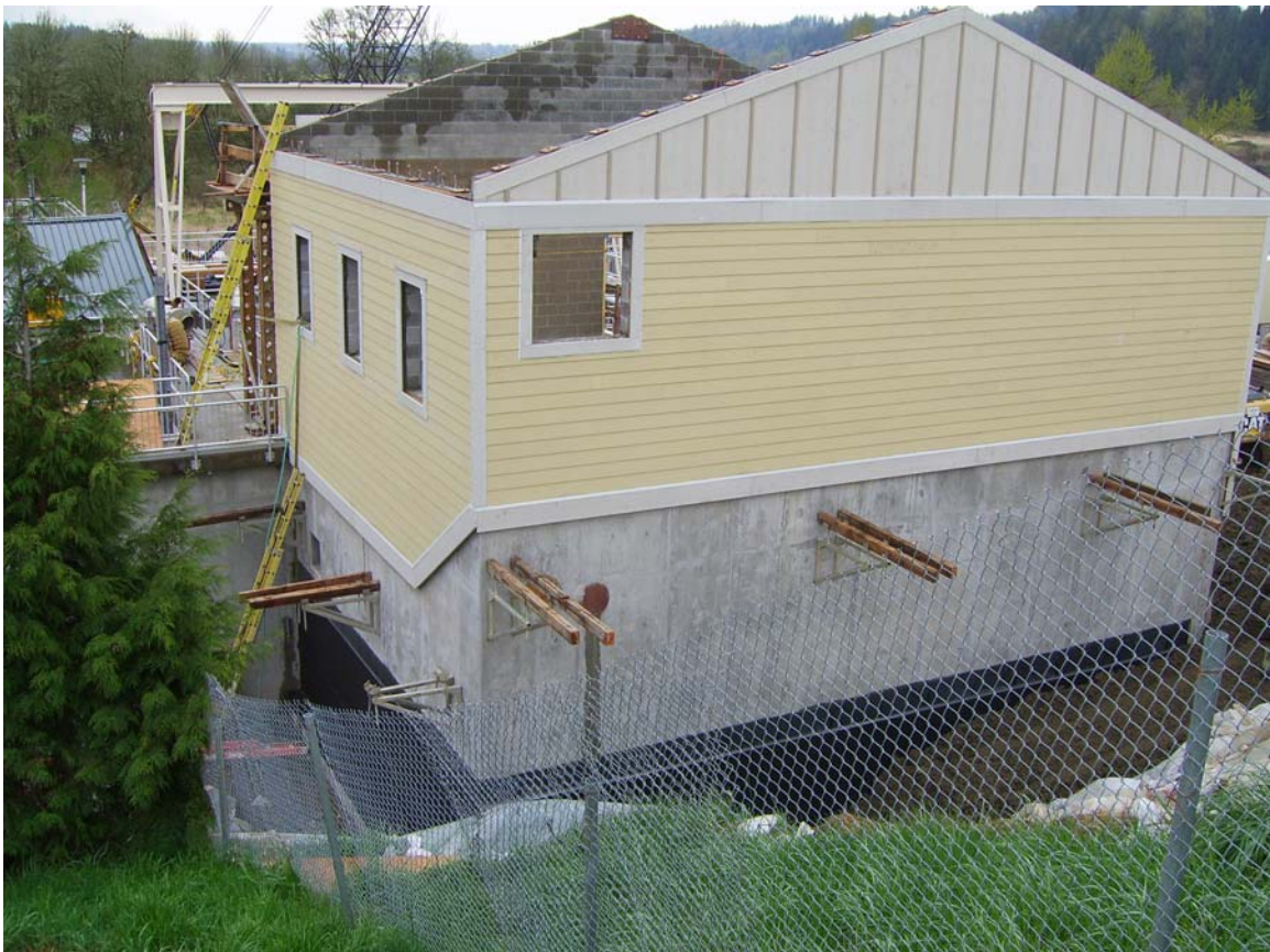
3/26/10 – Headworks building siding
