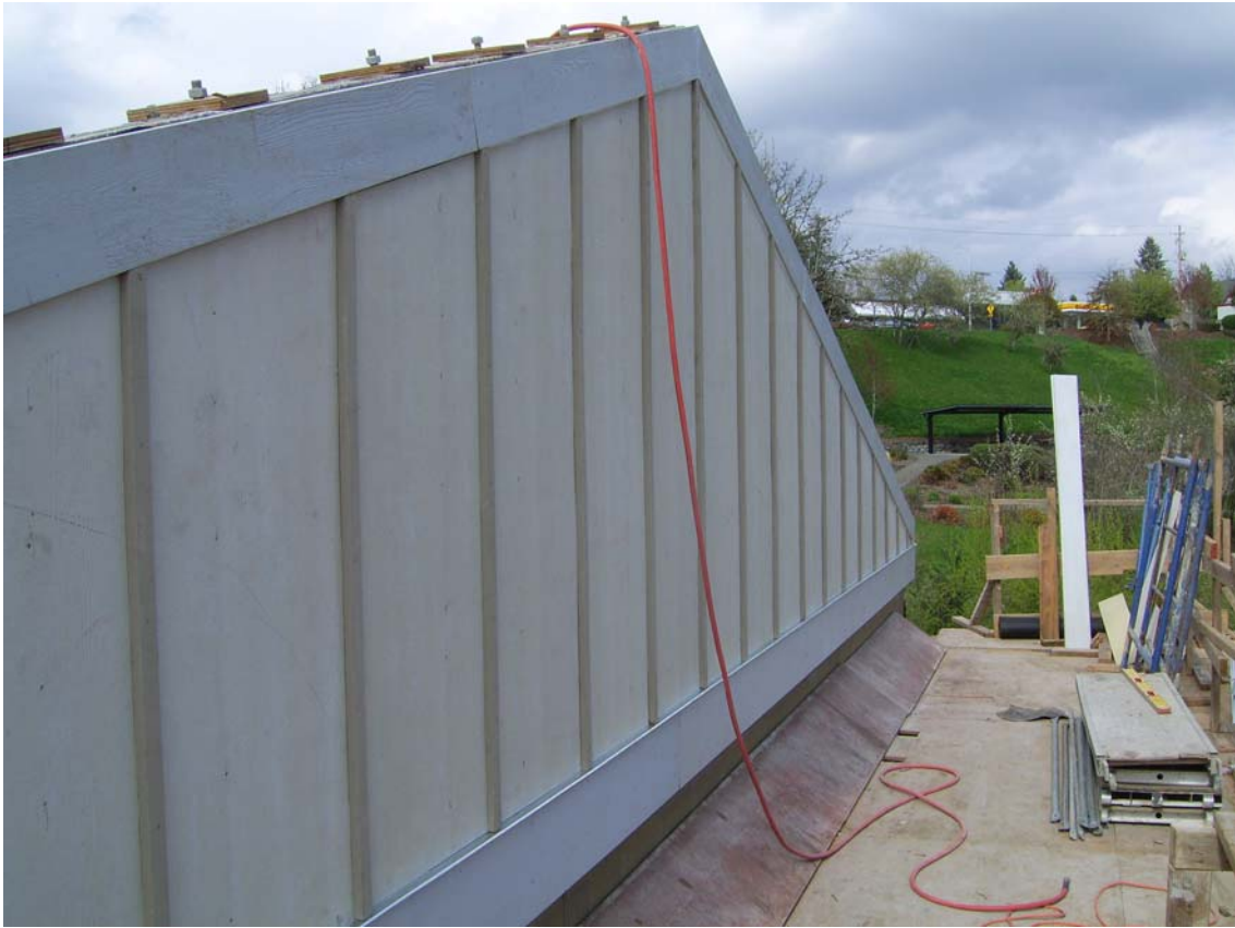
3/26/10 – Headworks siding on south gable end
