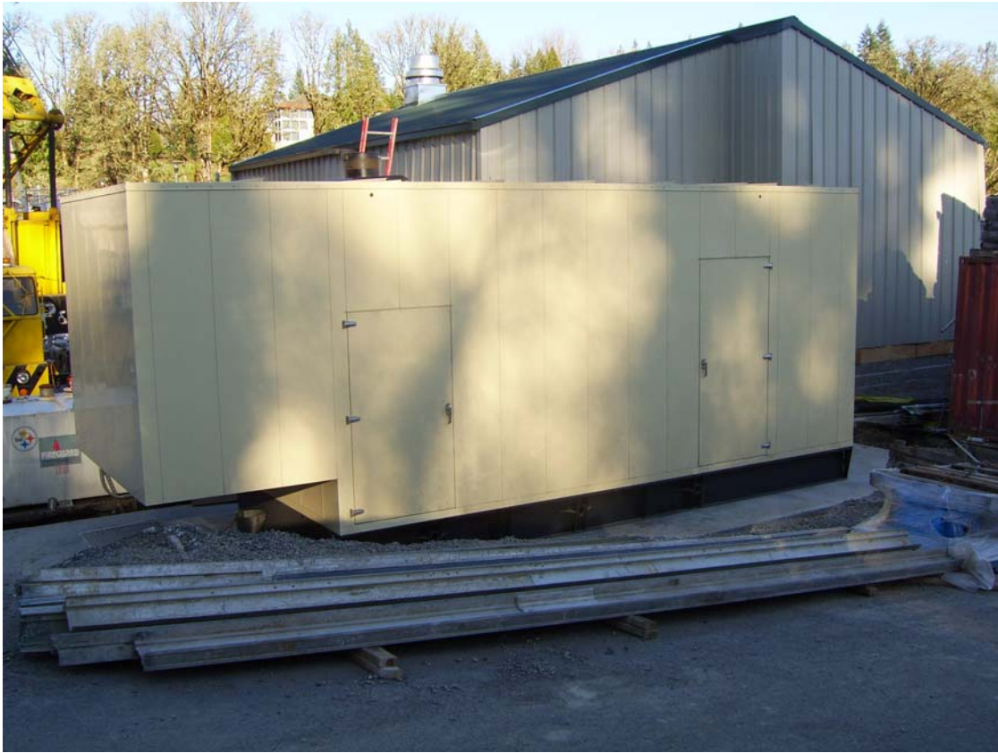
2/23/10 – 1,000 MW Generator on new concrete pad
