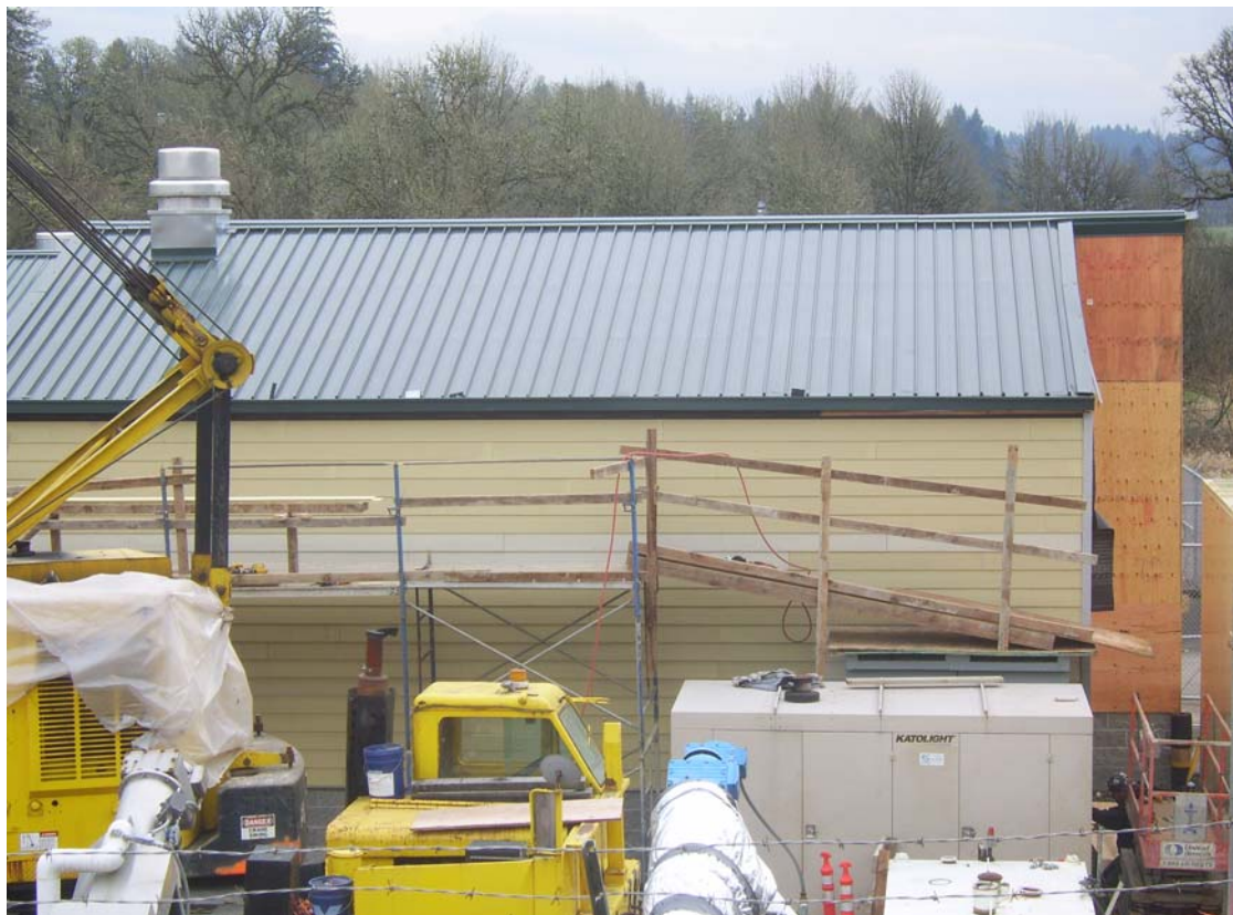
2/28/10 – New Control Room Siding Placement
