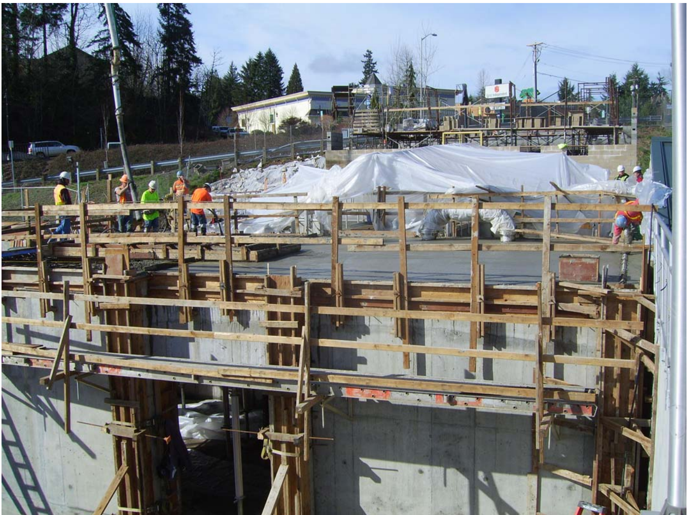
2/15/10 – Pouring Permeate Pump Room Lid Concrete
