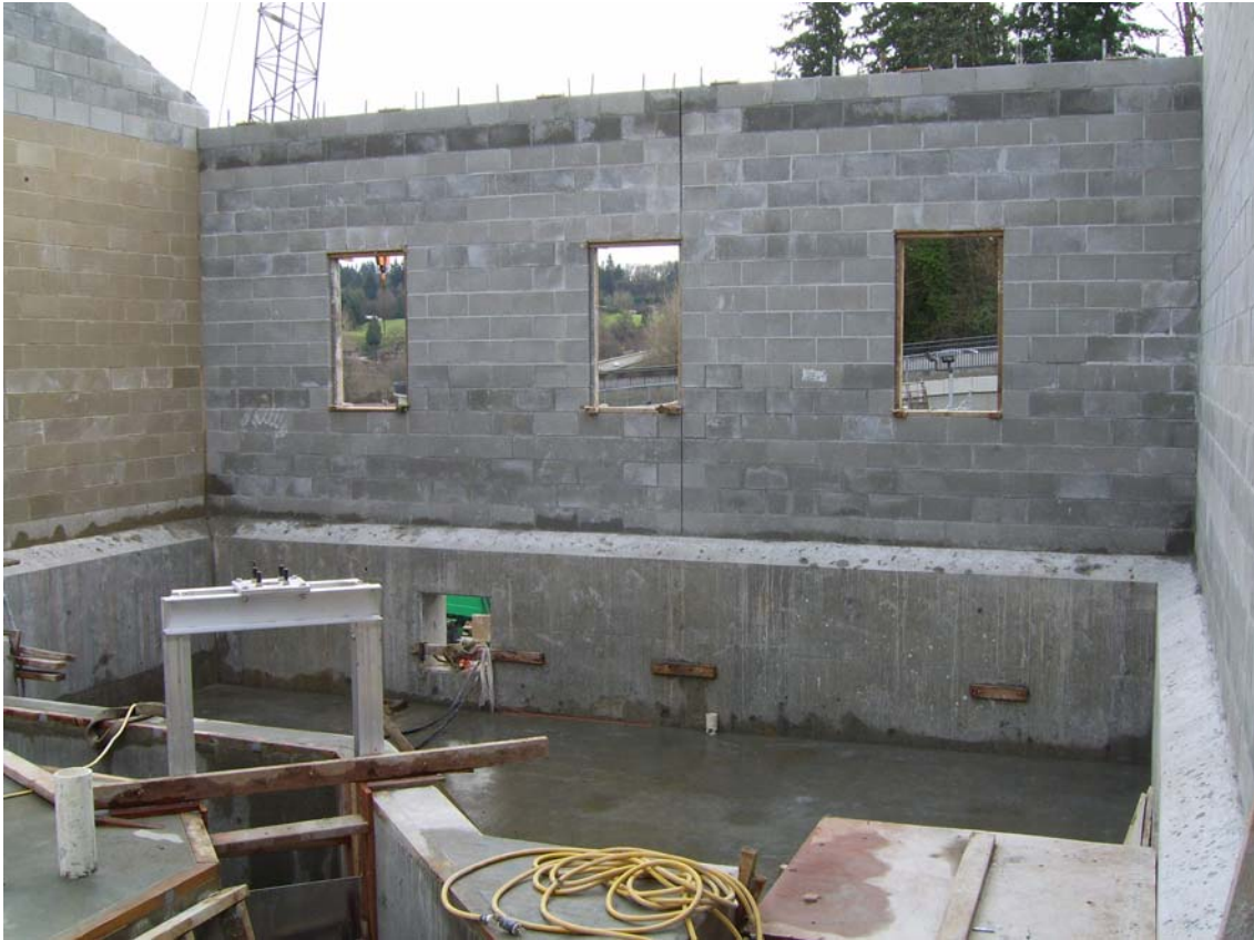
2/25/10 – Headworks Interior showing CMU walls and channel gate
